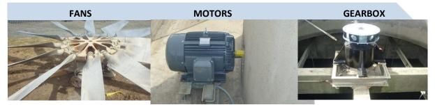
Four existing fans were replaced with FRP blades, HDG Hubs, Ductile Iron Hub Spools, and Aluminum Blade Clamps.
