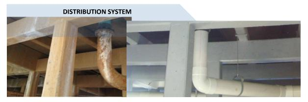
The existing distribution system piping comprised of schedule 40 steel and was seriously corroded. New schedule 40 PVC was used for headers and lateral distribution. ABS nozzles were installed for optimal flow and dispersion of spray system.
