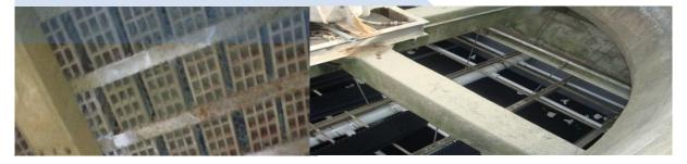
Existing fill was replaced with new PVC fill:15 mil after forming (Brentwood OF21ma-15). Drift eliminators were replaced with PVC Cellular 20 mil. FRP structural shapes were used for fill and drift eliminator support.
