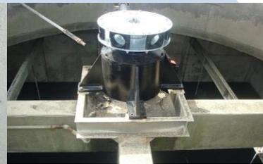
Four existing fans were replaced with FRP blades, HDG Hubs, Ductile Iron Hub Spools, and Aluminum Blade Clamps.
