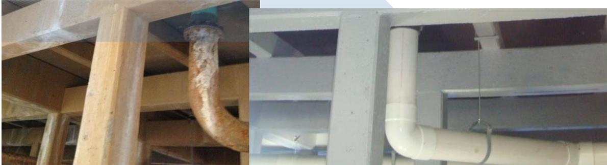
The existing distribution system piping comprised of schedule 40 steel and was seriously corroded. New schedule 40 PVC was used for headers and lateral distribution. ABS nozzles were installed for optimal flow and dispersion of spray system.
